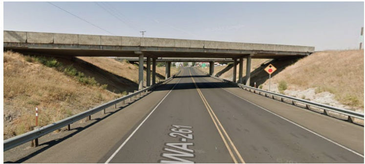
Figure 11. Northbound on SR 261 at I-90 Overcrossing
