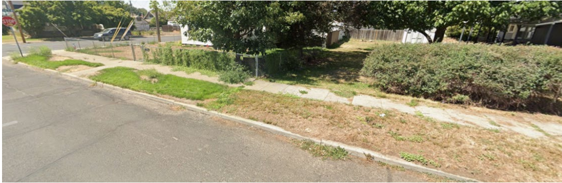
Figure 19. Sidewalk Obstruction on West Side of E 7th Avenue between Division and Columbia Streets
