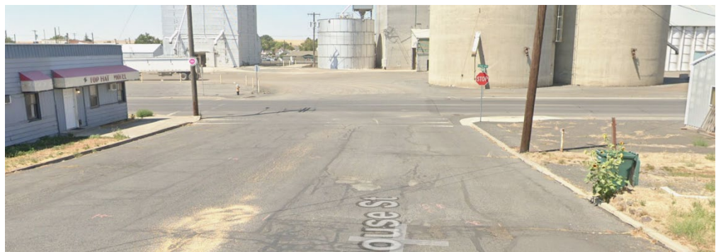
Figure 21. Sidewalk Ends on Palouse Street between 1st and 2nd Avenues
