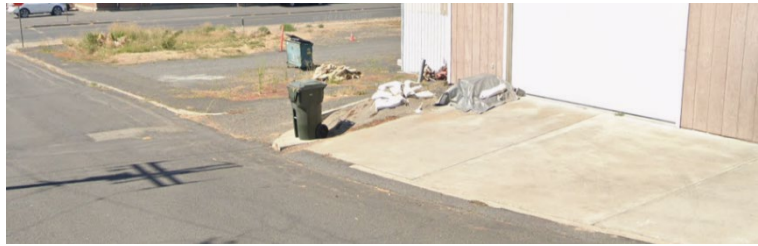
Figure 37. North Side of Columbia St between 1st and 2nd Avenues
