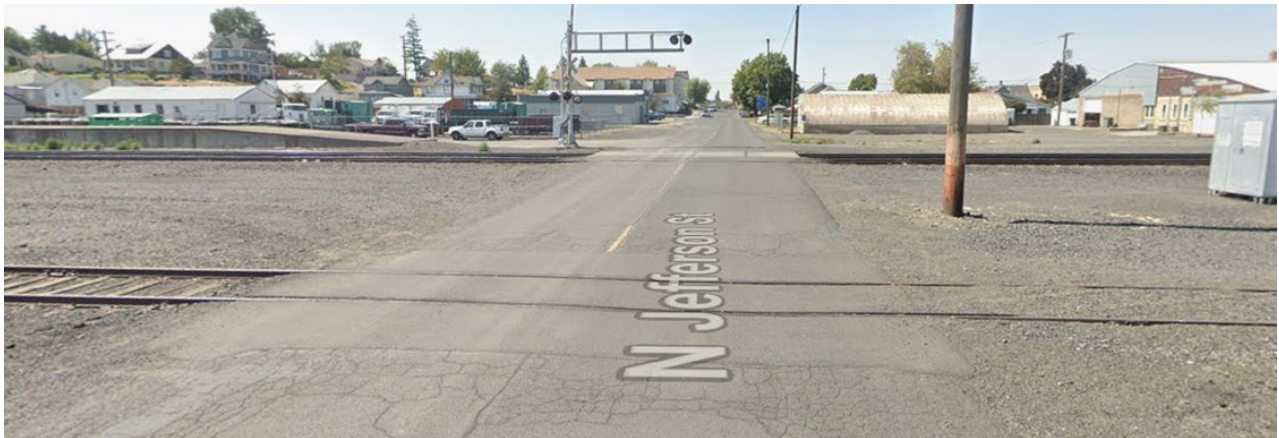
Figure 14. Northbound on Jefferson Street at BNSF Railroad and Spur Line Crossings
